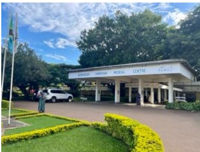
Image 1: KCMC main entrance
